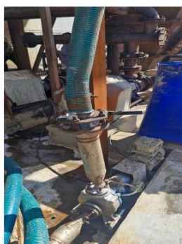
Location of Caustic lye leakage
